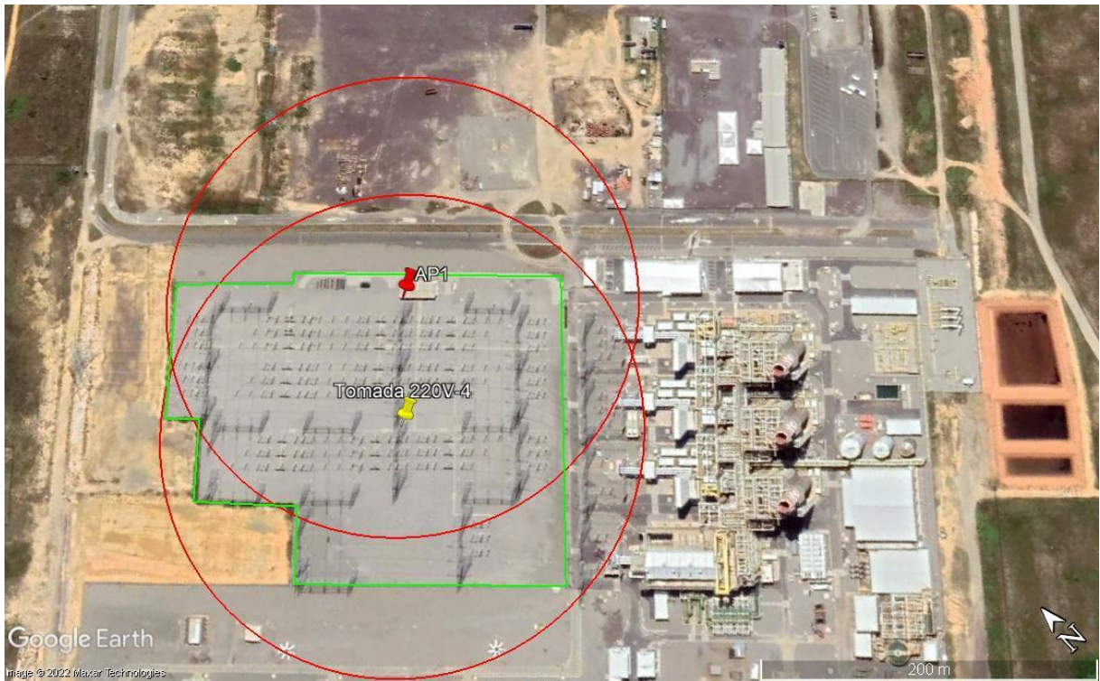
Figure 3.27: Mesh network coverage simulation in the substation of “UTE Porto de Sergipe I”.
